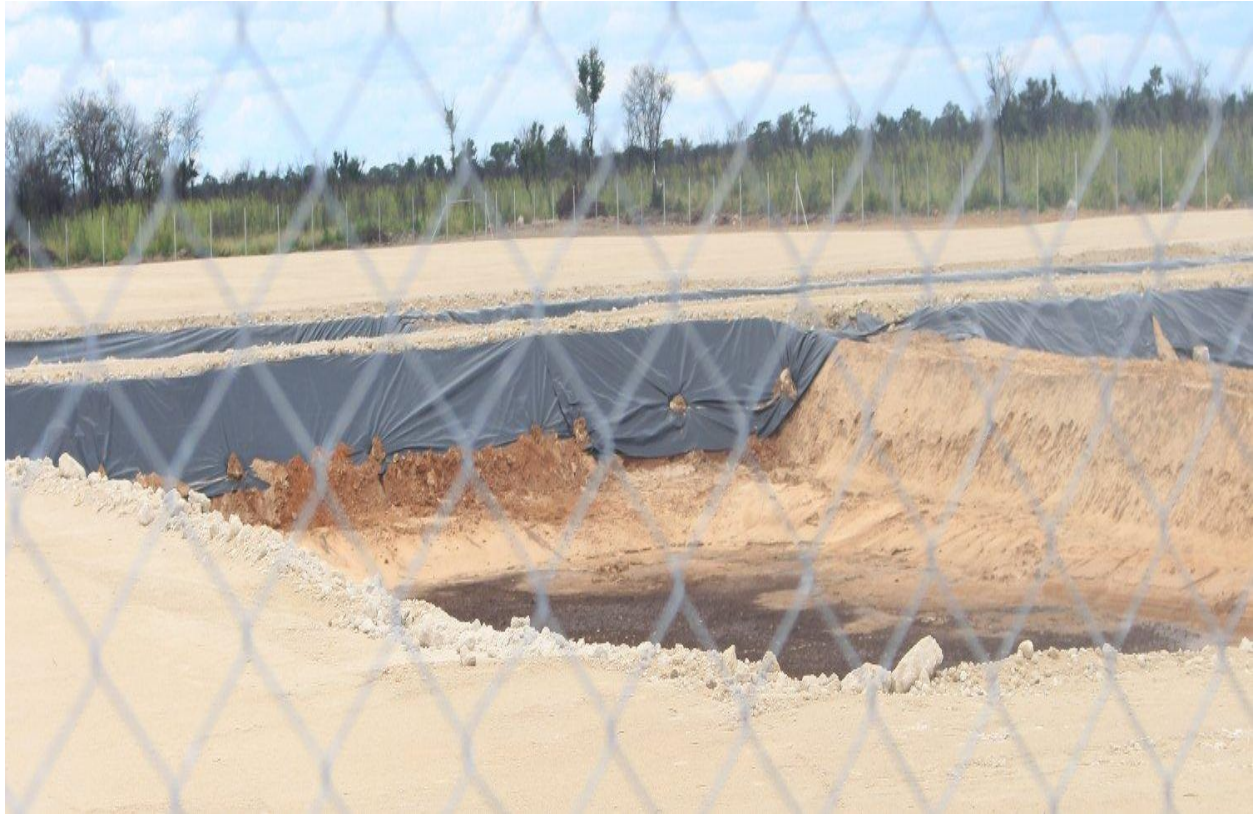
Mbambi, Unlined pit. March 2021.
